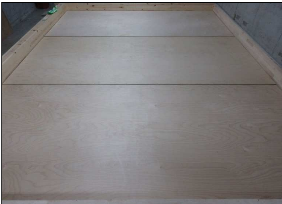
(c) Layout of the sound insulation panels
