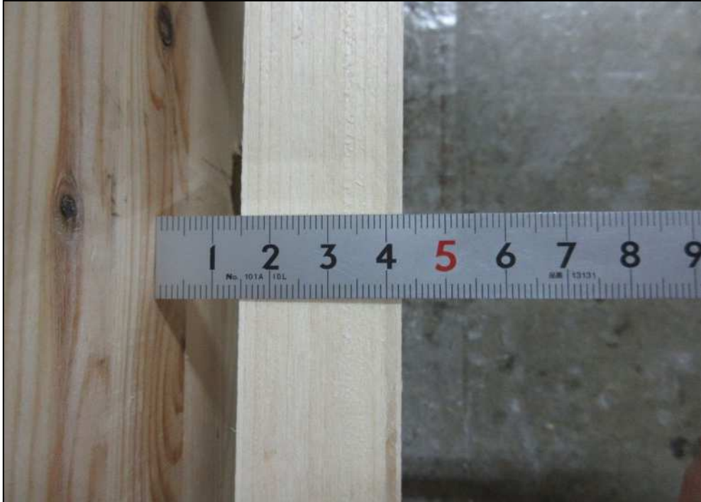
(a) Clearance of wooden perimeter joists
