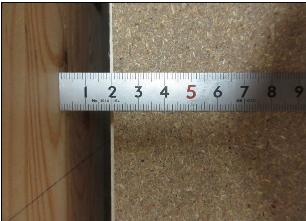
(b) Clearance of particle boards
