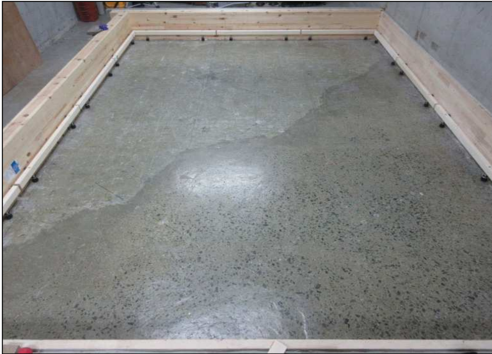
(a) Layout of wooden perimeter joists
